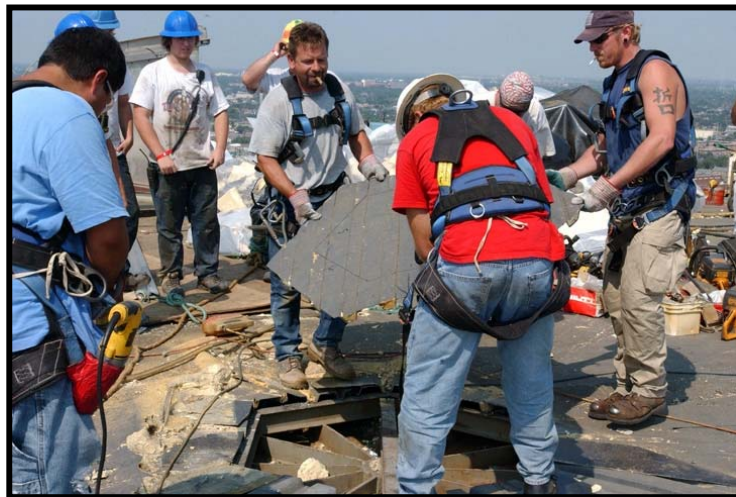
Left Photo: The final steel decking piece is placed on the Dome’s roof.
